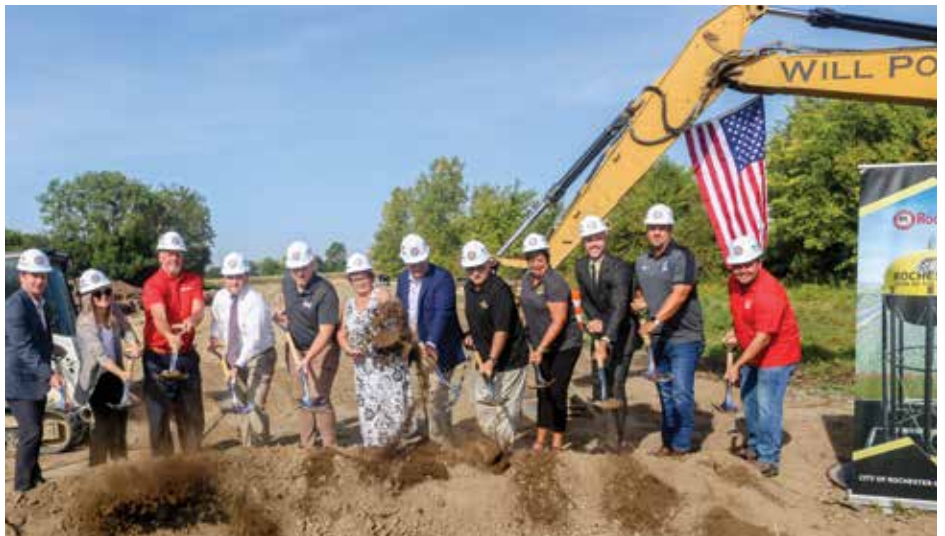
Groundbreaking for the $26 million Chamberlain Industrial Park. The site, located off of U.S. 31 and State Road 25 south of Rochester, provides a variety of economic opportunities for Fulton, Cass and Miami counties.
