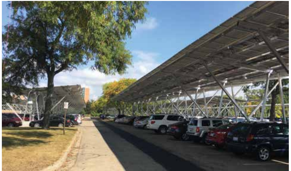
A solar carport covering more than 4,500 parking space at Michigan State University is one of 10 solar projects 1st Source Bank has invested in since late 2016.
