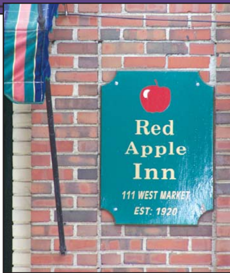
Following renovation, the former Red Apple Inn will offer modern conveniences to guests while retaining a historic feel.
