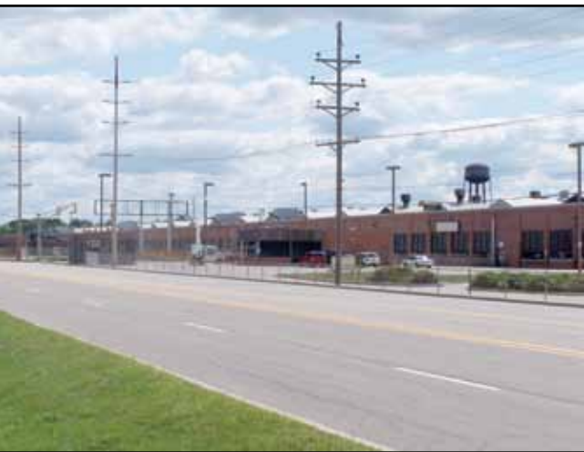
The now vacant BorgWarner facility is one example of Muncie's shift away from an automotive manufacturing hub. Plans call for the building to be redeveloped for multiple tenants.
