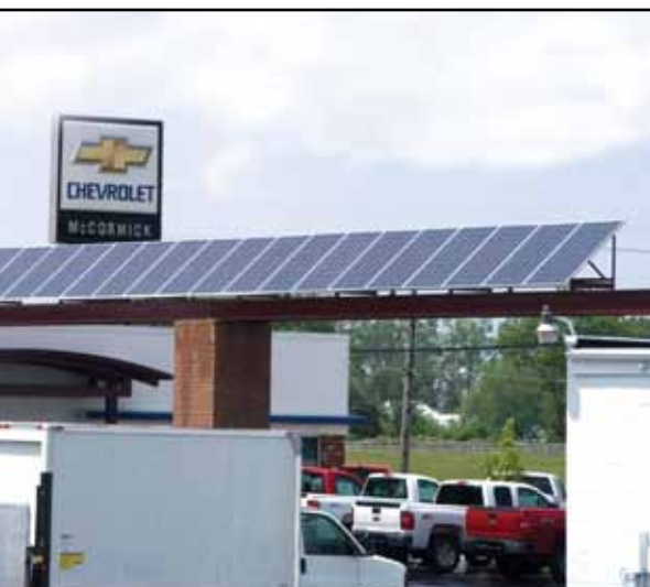
McCormick Motors' new solar panel is just one component of the Chevrolet dealer's multi-faceted effort to minimize energy consumption.
