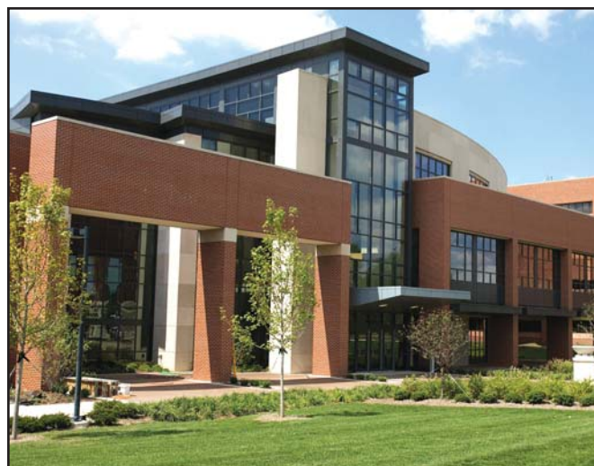
The David Letterman Communication and Media Building on Ball State's campus is filled with "LEEDing-edge" technology. The building is also a model of sustainability and reflects the university's strategic plan, which states that all new buildings will be LEED-certified at the silver rating or higher.
