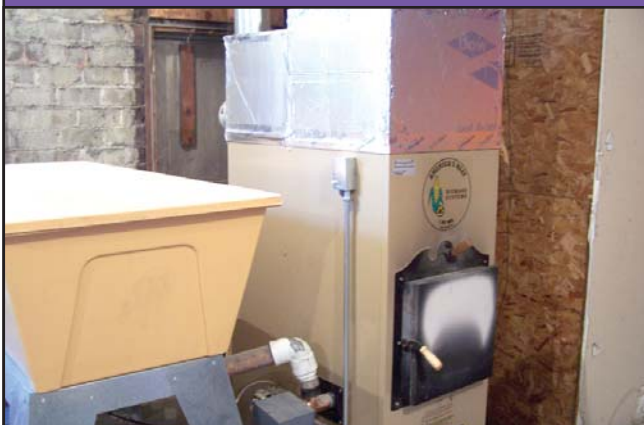
Corn feeds from a large vat into the furnace to produce heat.
